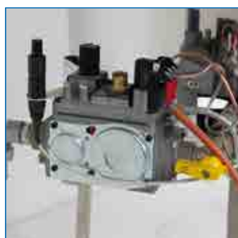
Valvola Termopila
